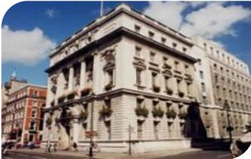
3 Whitehall Place is a Grade II listed building built by the Ministry of Works in 1951/52 as an extension to 55 Whitehall. The building is five storeys high with a set-back attic storey. The building was completely renovated in 2003/04 with the original façade retained and restored.
